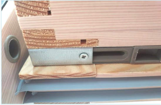
WINDOW UNBLOCKED - - the latch is hidden
